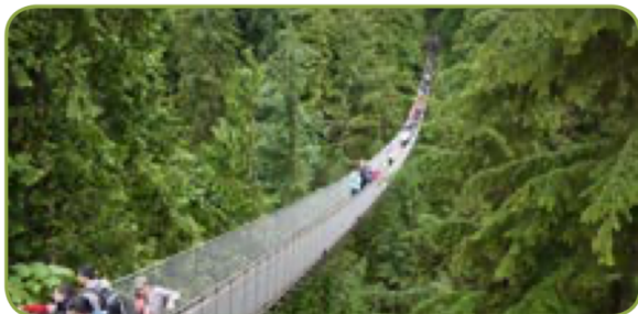
Capilano Suspension Bridge Vancouver
